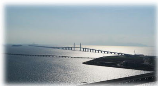
Ponte Hong Kong-Zhuhai-Macau
